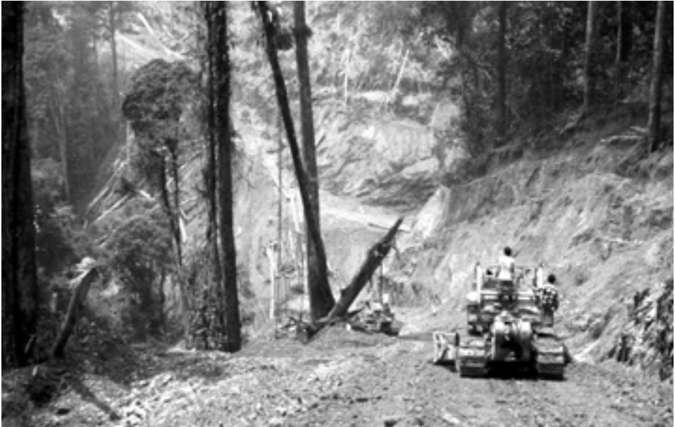
Figure 22. Logging roads are often poorly engineered unnecessarily wide, increasing forest fragmentation and a range of negative impacts. (Photo by Rob Fimbel)
